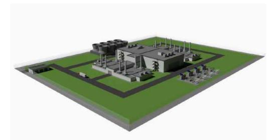
Figure 2.1: Layout of 4 SEALER-UK unit plant [Published with permission from LeadCold]
